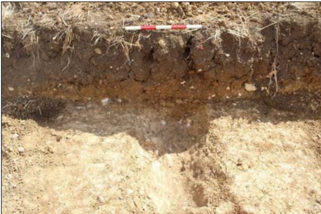
Plate 29: Gully [94206], looking east
